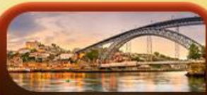
DOM LUIS I BRIDGE
